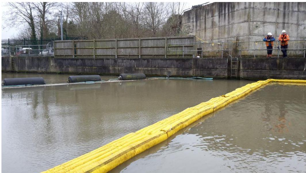
Oil Boom at Taplow, showing sections coupled together to span a larger river
